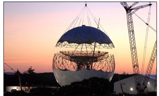
*Radome cap lift in May 2010 was one of the first steps in the HUSIR integration sequence. The HUSIR has increased W-band resolution while maintaining X-band sensitivity.*
